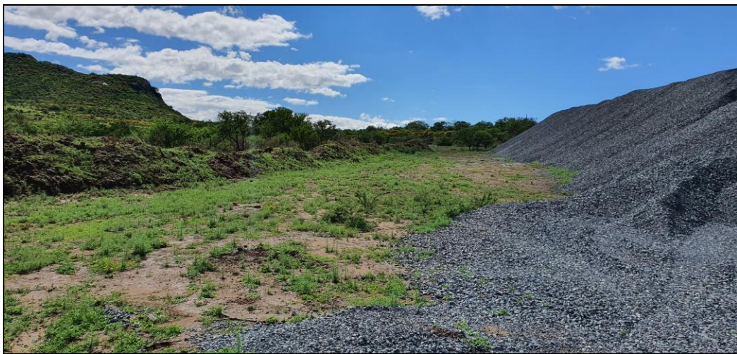
Figure 14: General view of the edge of the stockpiles in the mining footprint
