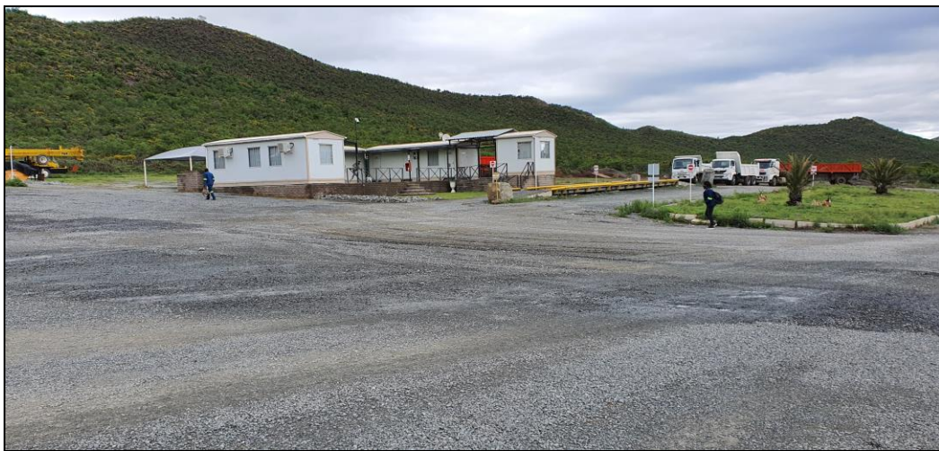
Figure 11: General view of the offices and associated infrastructure
